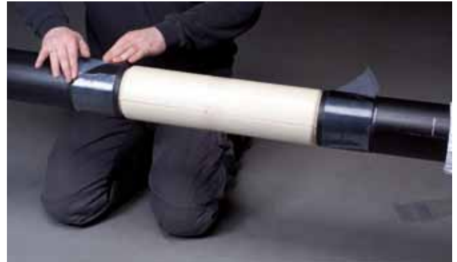
5.6 Wrap outwards the upper release liner on both sides in a 45 ° angle that the beginning of the film of both melting adhesive strips protrudes over the marking of the center distance.
