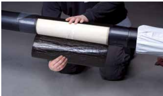
6.1 Remove the release liner at the bottom of the casing shrink film. Center the film over the PUR- insulation sleeve in a 90 °C angle to the pipe axis and wrap closely around the PUR –insulation sleeves. A sufficient overlap of the shrink film of at least 10 cm is important. On both ends the shrink film must overlap the casing pipes with at least 2.5 cm.
