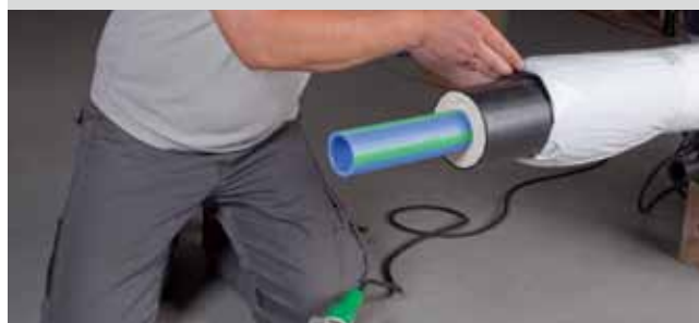
At the stop of the peeling tool the barrier layer is removed up to the welding depth. Now the tool can be pulled off.
