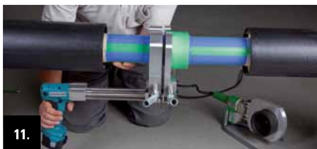
11. Press the pipe end, within the processing time, with the welding jig up to the end of the welding depth in the welding socket.
