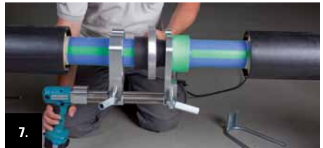
7. Position the manual welding device in the center of fitting and pipe end and drive together the welding jig slowly.
