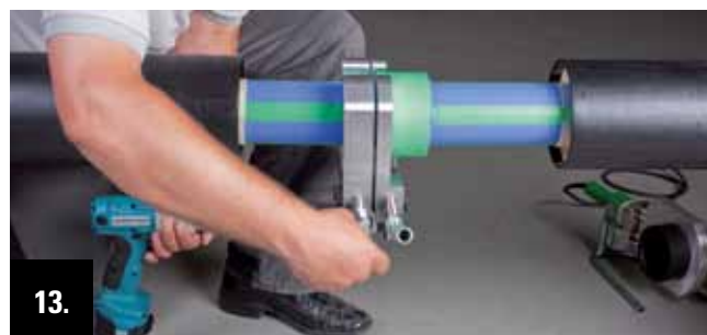
13. After the cooling time release the clamping jaws on the pipe side by unscrewing the fixing screw.
